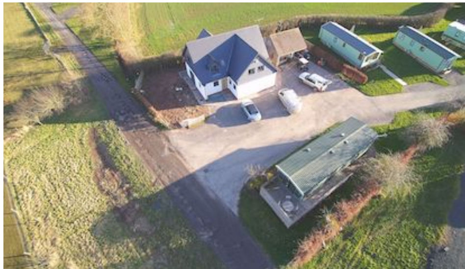
An aerial shot of Brian and Sandra's new house at St Michaels, taken by builder Chris Steventon
